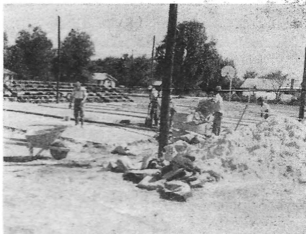
The erection of cement courts and lighting get on the way.
